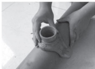
4. Install the Mechanical Tee in the hole.
